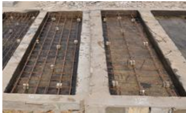
Fig 1 Reinforcement details of SV1 & SV2
